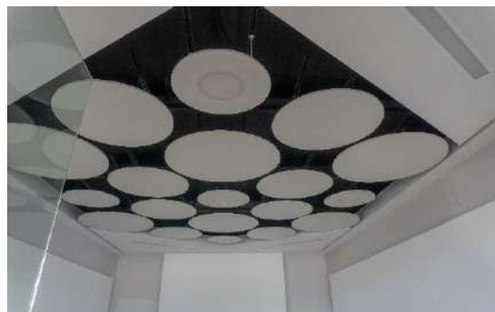
Cielo Raso local FF12
