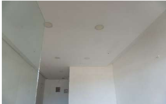
Cielo Raso Local FF10
