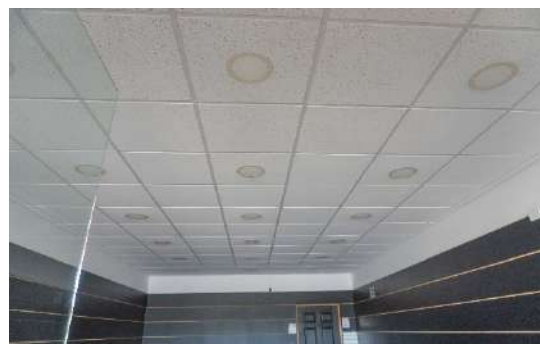
Cielo Raso local FF11
