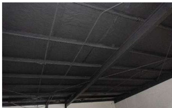
Cielo Raso Local FF15
