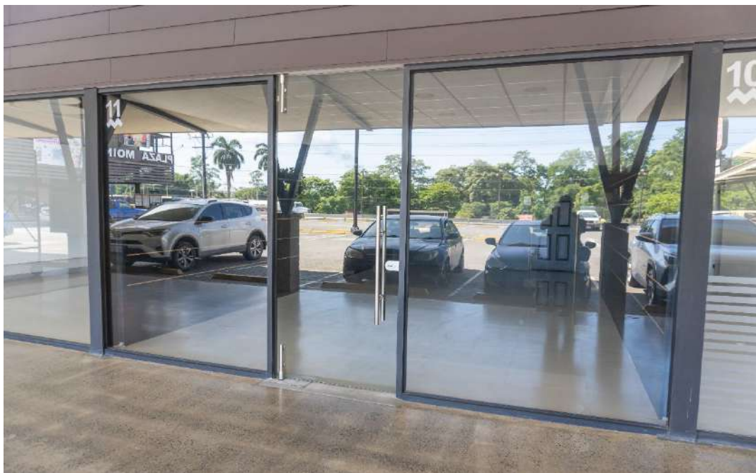
Fachada Frontal Local FF11
