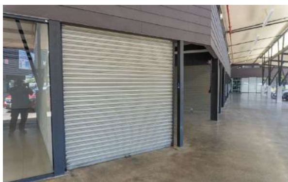
Fachada Frontal Local K-3 (Bodega)
